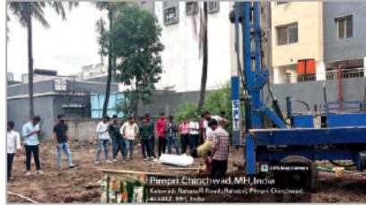
Study of building Foundation
