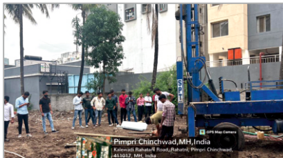
Study of building Foundation
